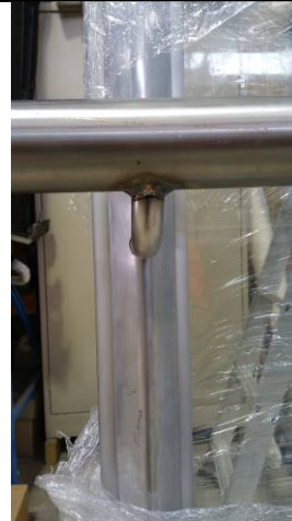
Photo 12 Hand Rail Loading Outwards & Downwards - Welded to Stainless Steel Bracket
